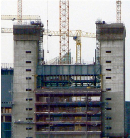
The tower before the roof was raised
