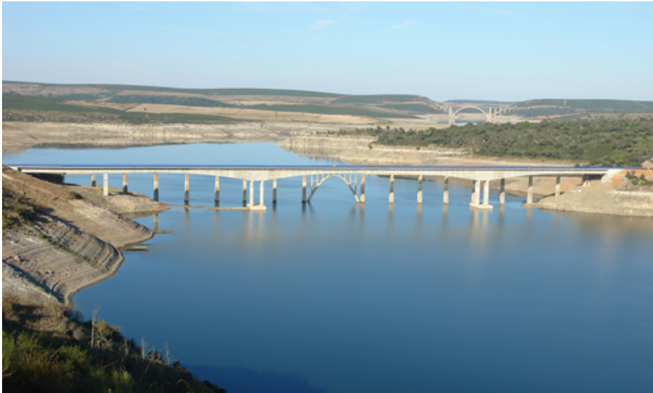
View of the El Manzanal bridge
